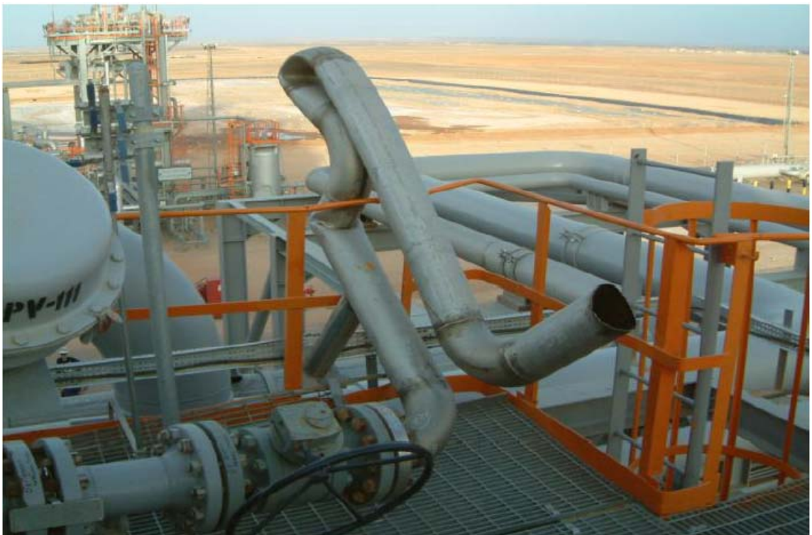
Figure 4 – Reaction Force Example – Failure of Unsupported Piping
