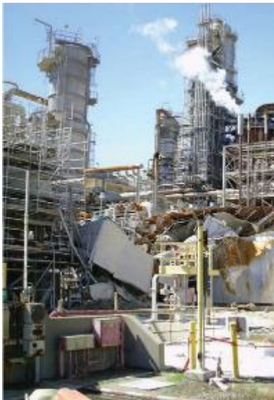
Figure 10: ExxonMobil Torrance Refinery explosion Feb 2015
