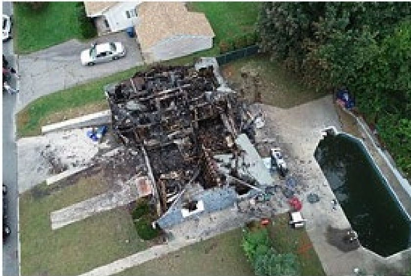
Figure 1: Merrimack Valley MA, Gas construction incident – Sept 2018
