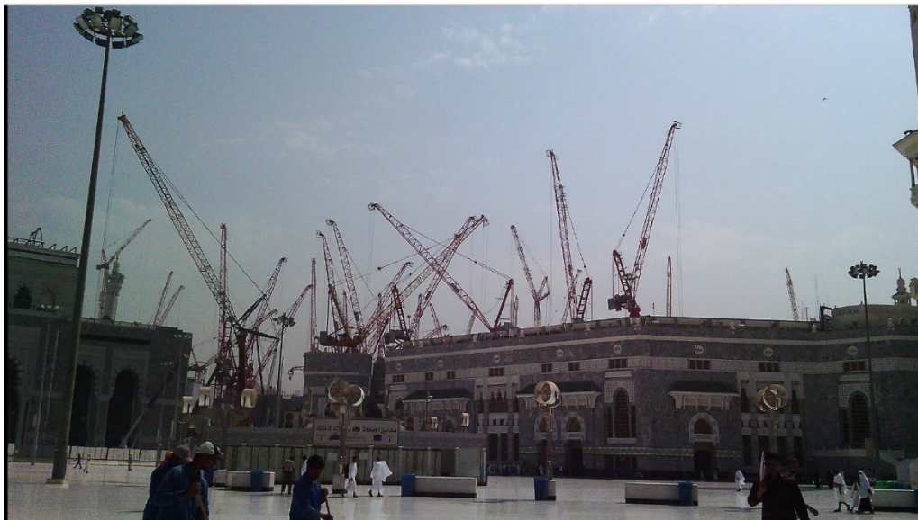
Figure 11: Cranes Similar to those used in Mecca, Saudi Arabia Incident 2015
