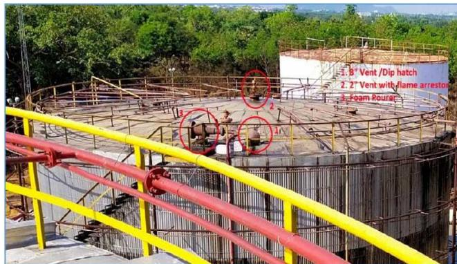
In general, it is not practical to provide adequate relief for large low pressure monomer storage tanks under either a process induced runaway condition or a fire induced runaway condition.
