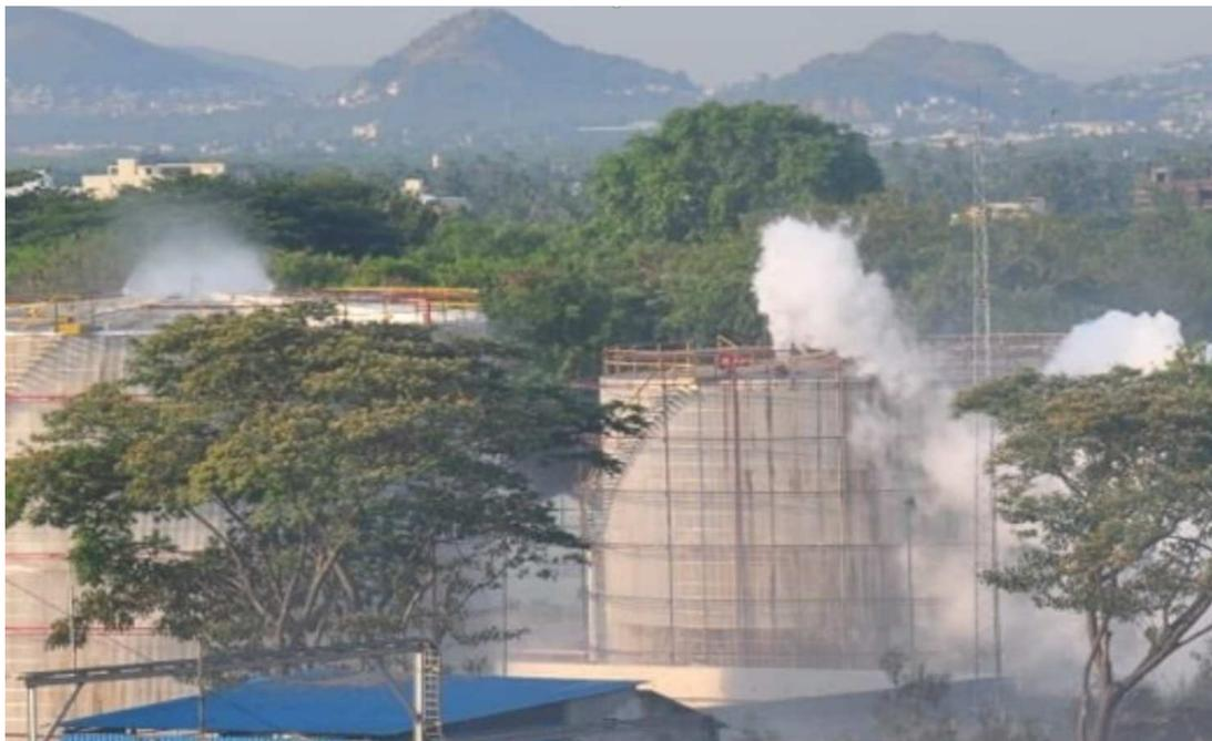
The refrigeration unit may have been shut down the day the plant was closed due to the COVID-19 lockdown. It was also reported that there may have been a malfunction of the temperature controls for the bottom of the tank and that the bottom of the tank was still at 17 C until the incident occurred [15].
