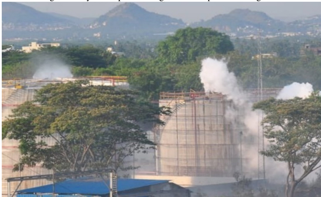
Figure 3: Styrene vapors leaking from the top of the storage tank
